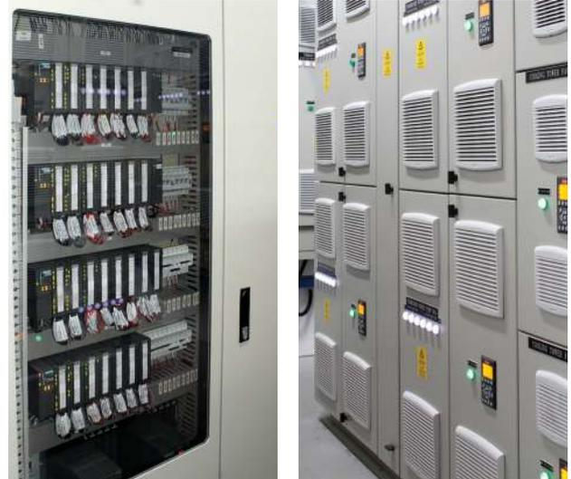
Instrumentation panels enable the remote monitoring and control of the air-conditioning system.
