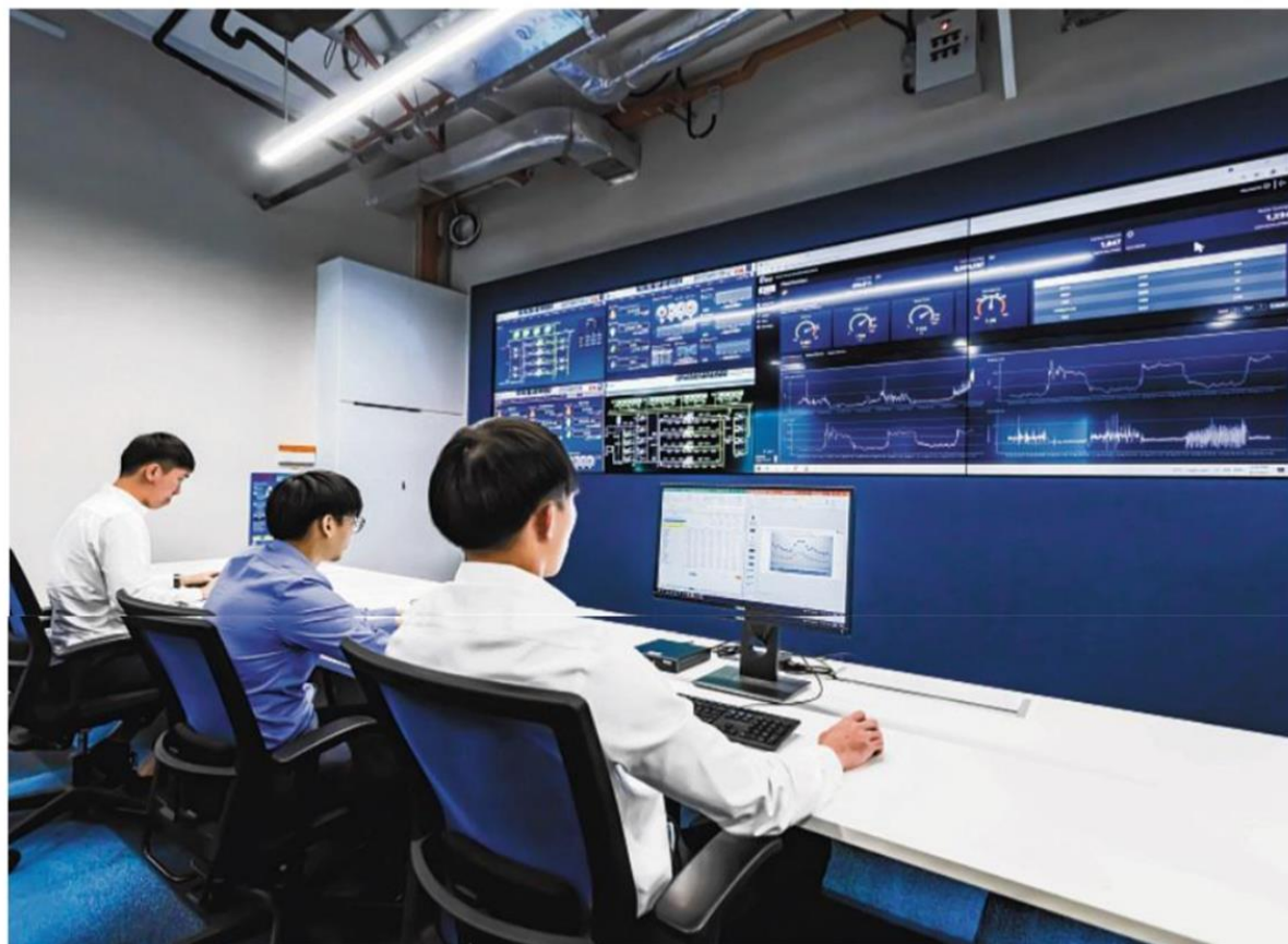
BBP helps clients save their electricity bill by using its patented software and data analytics to optimise the amount of energy they need to cool their facilities. PHOTO: BARGHEST BUILDING PERFORMANCE
